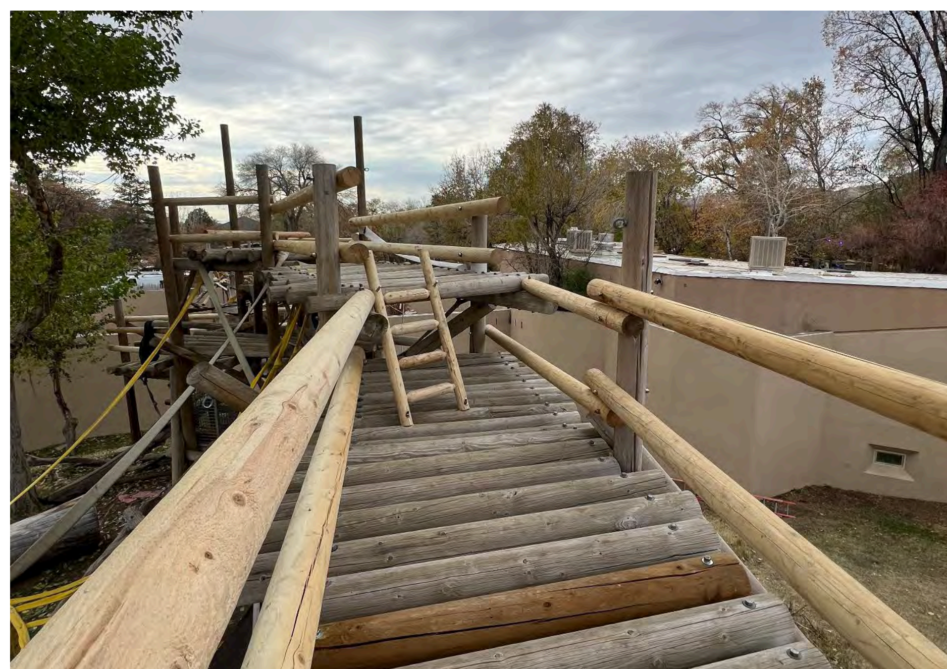
Completed construction of guardrail and ladder system
